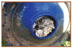
Ragged pump before installation of DERAGGER II
